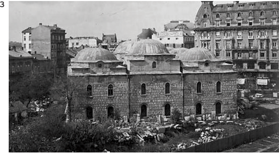
1-3. Sofia, Mahmud Pasha Mosque in old photographs. The second photo shows remains of a five-bayed portico prior to the construction of the present historicizing entrance structure shown on the first photo. The third photo shows the exterior of the mihrab wall, now enveloped by a modern building. The accentuation of the longitudinal axis through an elevation of its three domed bays is visible on all three photos.
